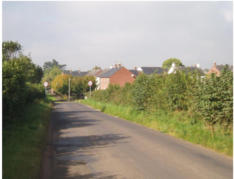
View toward Lower Broomhedge on Lurganure Road with the Gallop's Housing Development on right
