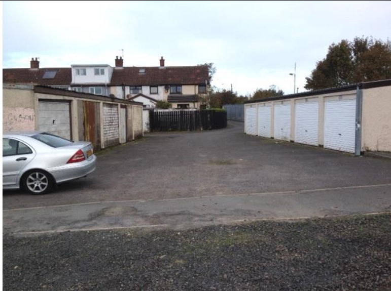
Lock-up garages adjacent WwTW
